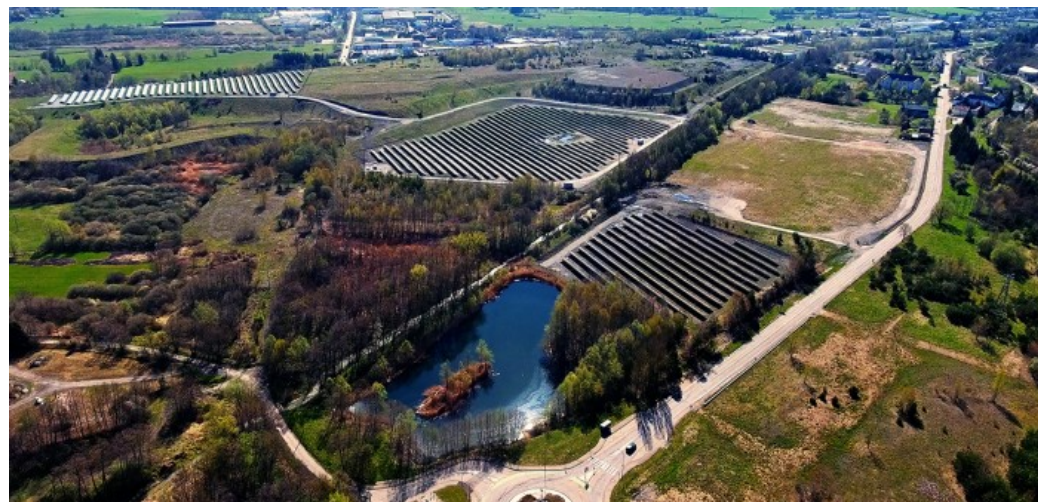
Centrale photovoltaïque Susville
